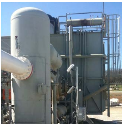
Bullhorn SDT16-SAT installation on a compressor
